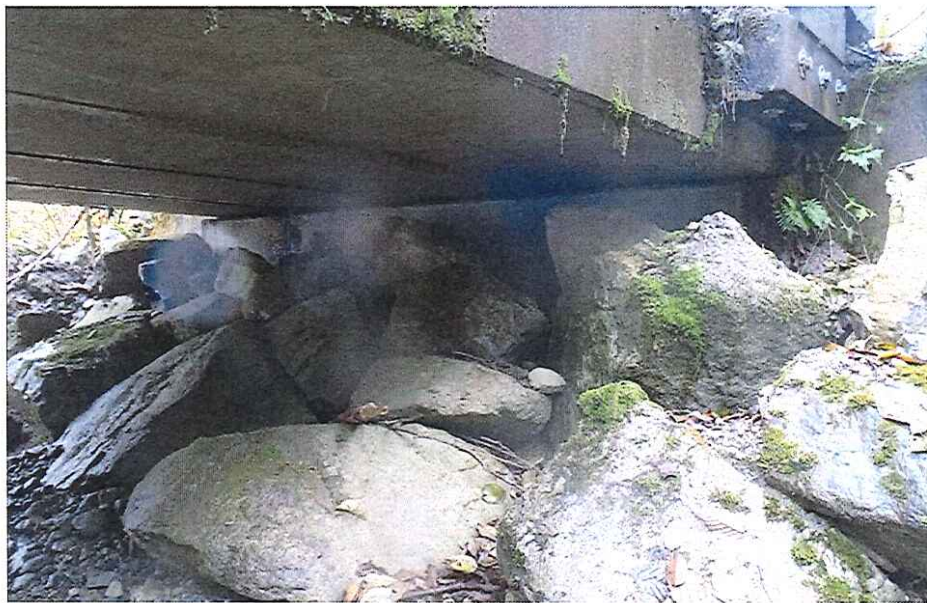
CK2417 Right Abutment
