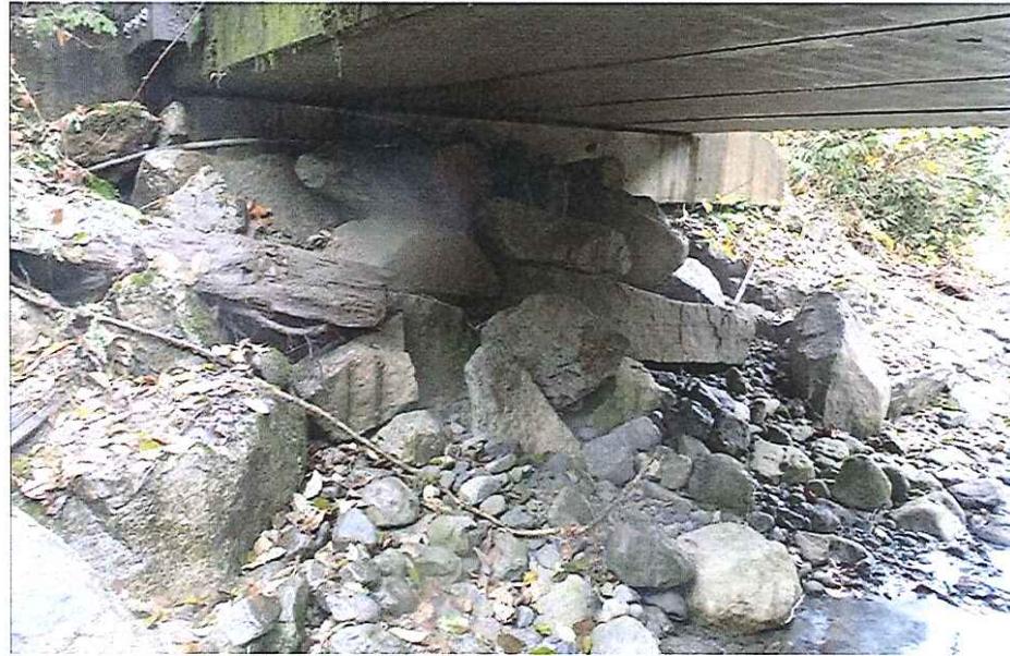
CK2417 Left Abutment
